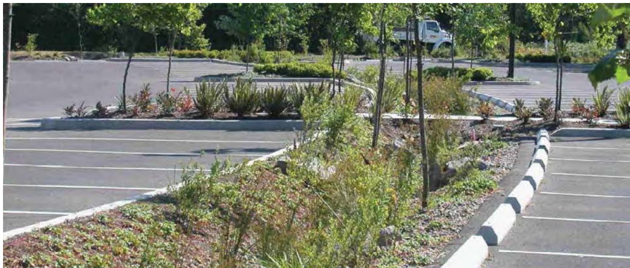
Figure 5-7 Example of Bioretention Facility
