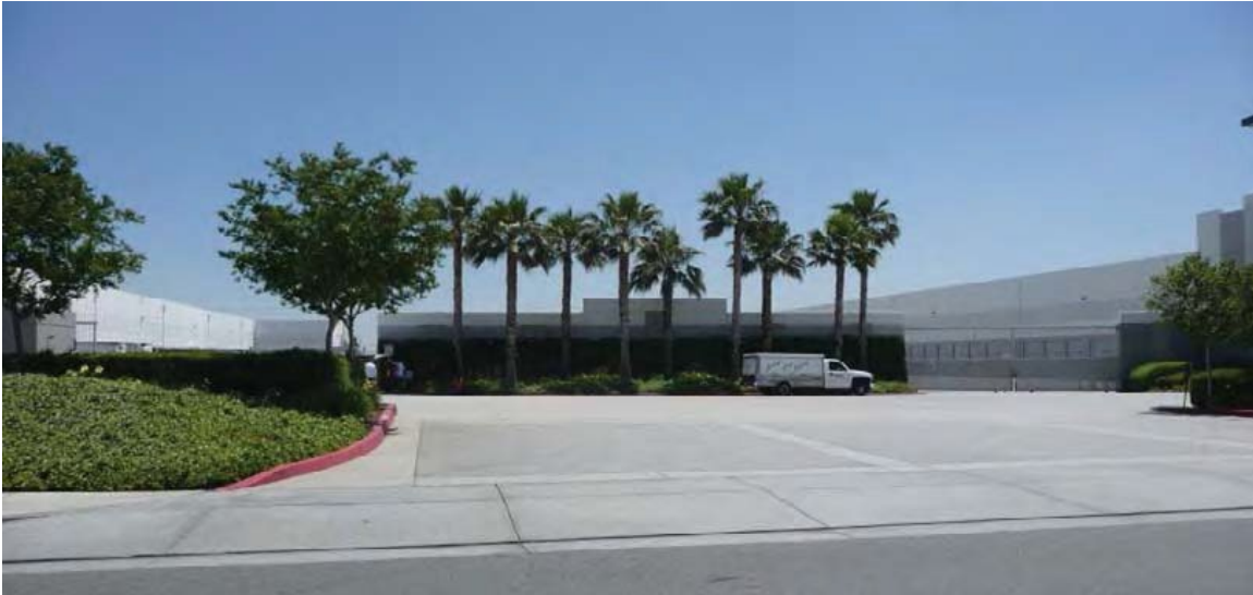
Figure 5-25 Example of Appropriate Ground Mounted Equipment Screening
