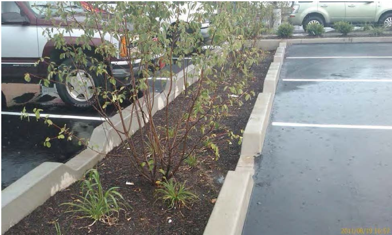
Figure 5-35 Example of Bio-swale
